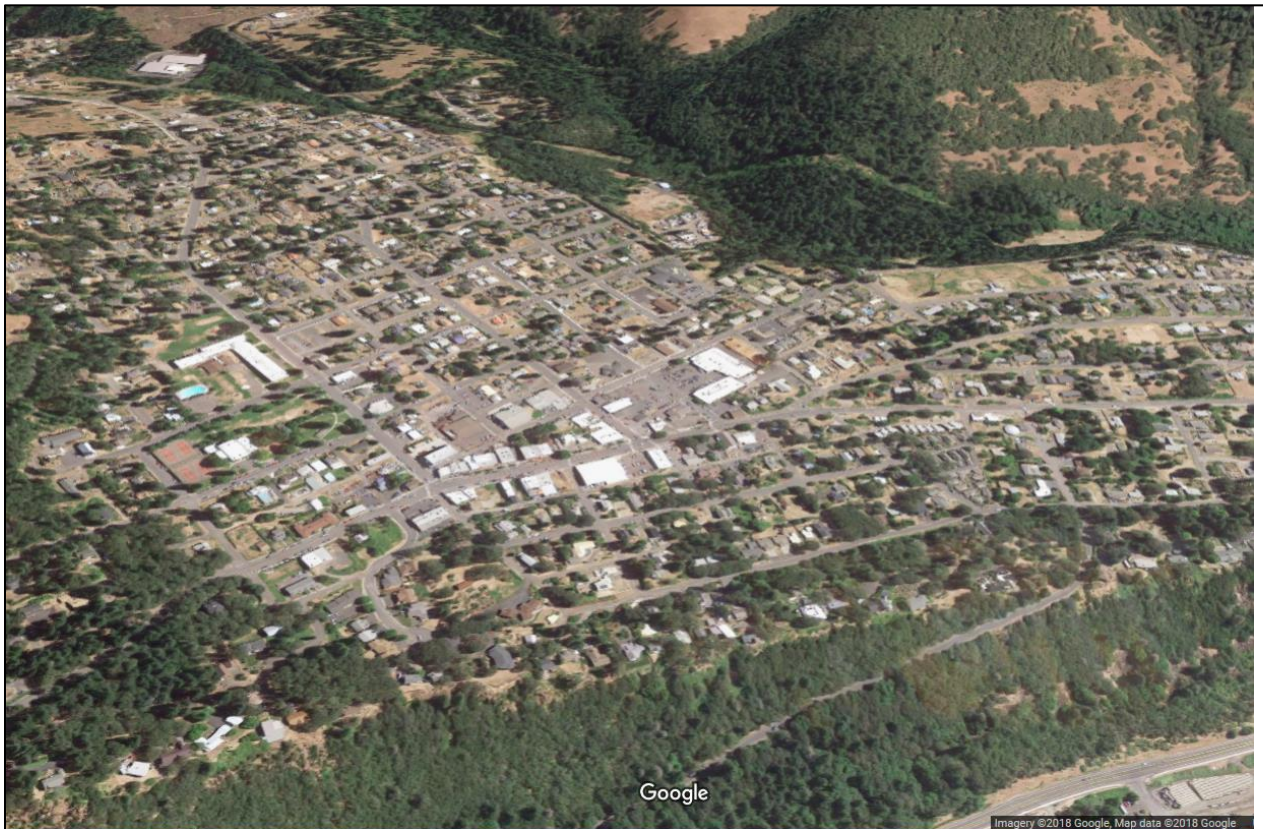
Figure 1. City of White Salmon aerial view.
